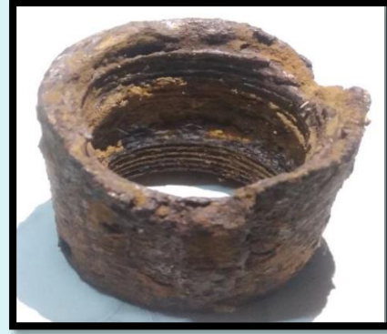
Failure piece of CI joint
